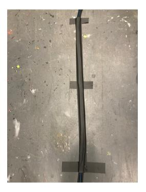
Run a piece of tape along each side of the centered piece of tape to cover the entire width of the cable run. If you have a wide area to cover, repeat this until completely covered
