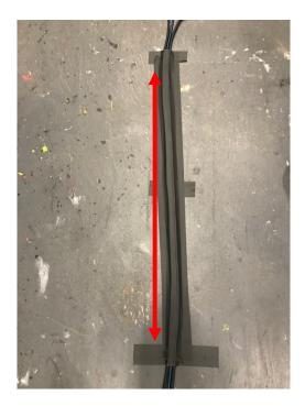
Once the cable width is covered, attach a few pieces of spike tape to ensure people are able to see it in low light. The finished product should look like the image below
