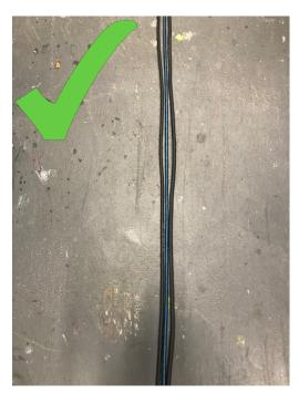
• Attach a few small pieces of tape along the entire cable run to secure the cables in place. Then run a piece of tape directly down the center
